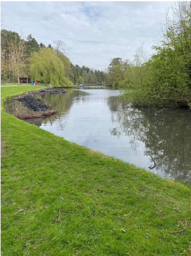
Figure 2.14. Brush berms being created along the Lake margin
