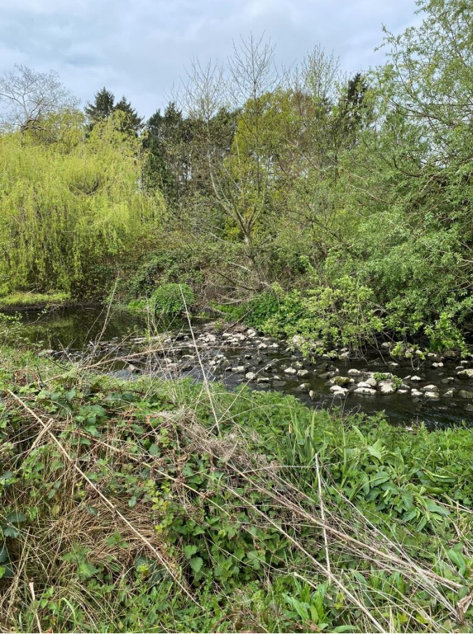
Figure 2.6. Rock ramp showing composition along the River Blythe at Brueton Park
