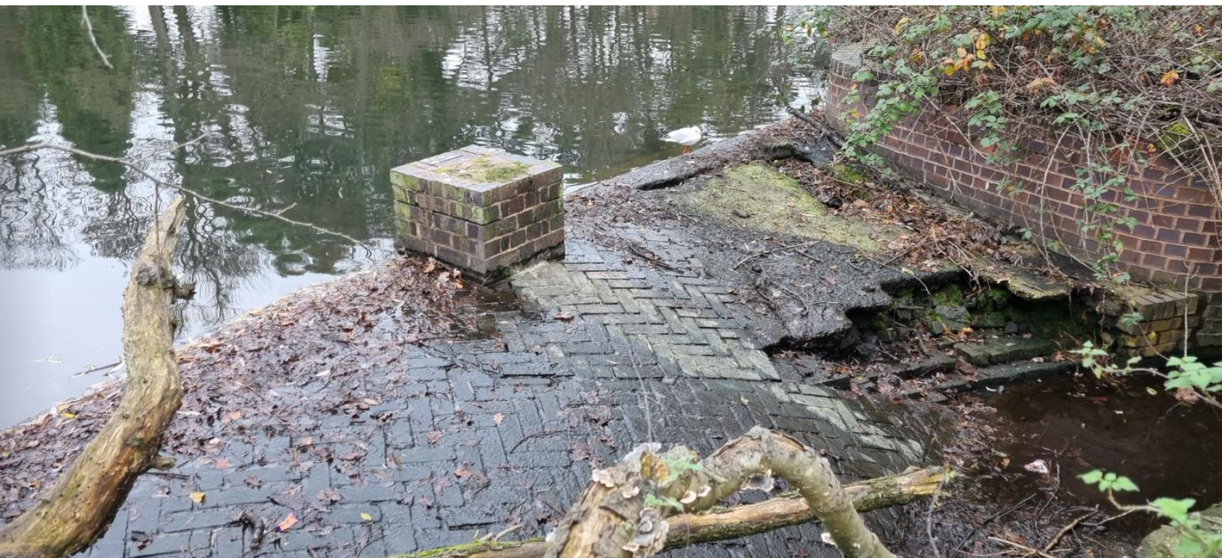
Figure 2.7. Side weir structure
