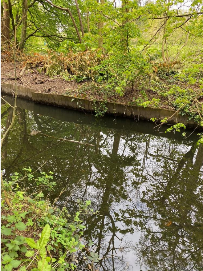
Figure 2.12. Ad hoc bank protection on the left bank island between the main watercourse and the Lake
